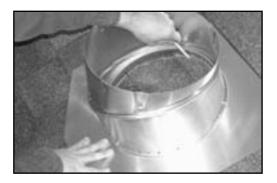
3. Locate base opening between rafters and mark hole(s) to be cut. Locate rafters by tapping roof.
