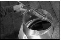
8.Seal the adjusting seam and the base/elbow connection seam on inside with roofing cement. Seal locking clamp holes and all exposed nails with roofing cement.
