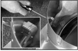
7.Place locking clamp across seam and tighten as shown, with included screw.
