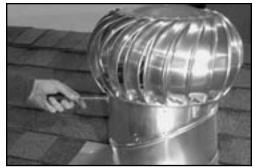
9.Position whirlybird on the base. Line up the predrilled holes in the brackets and elbow and fasten with sheet metal screws.
