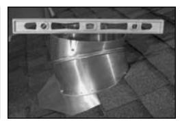
6.Rotate top of elbow to level position by turning counter clockwise.
